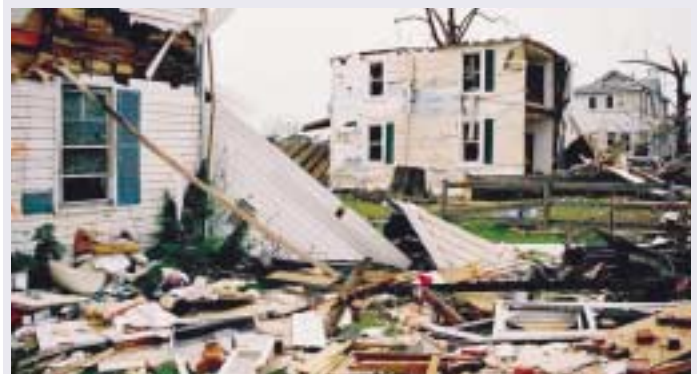
Condemned homes, shattered by the April 28, tornado stand abandoned along Oak avenue in La Plata along with stripped or felled trees. Generally they simply stand empty and abandoned until demolished.
